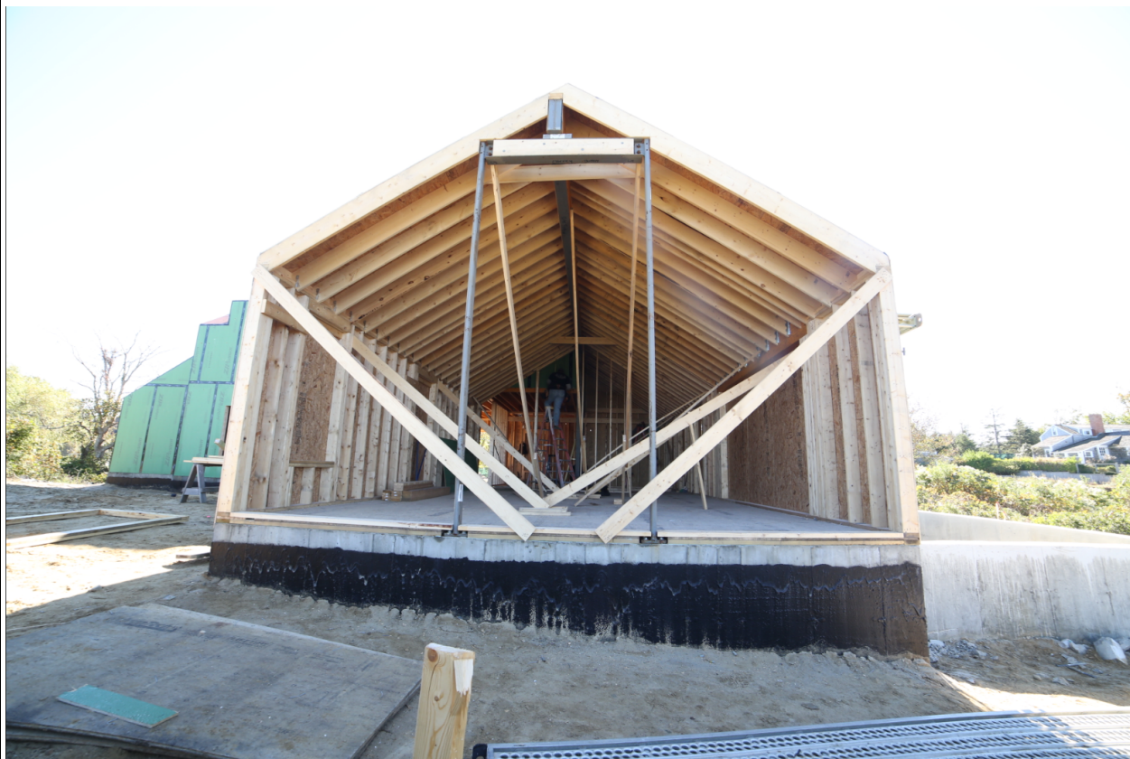
Offset ridge beam and interrupted load path at guest house
